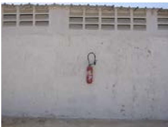
An extinguisher must be placed on the wall outside the storeroom. (Photo B. Schiffers)
