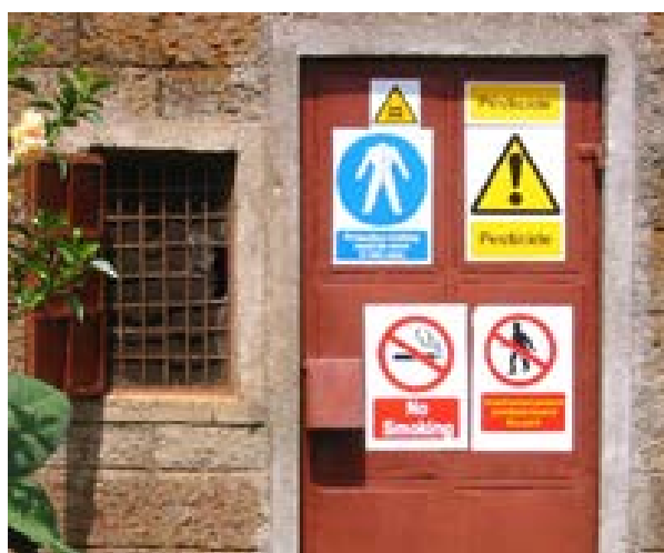
Example of protected access: grate on the window, door locked and/or padlocked.
