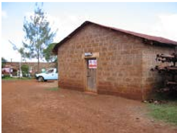
Example of a product storeroom in Kenya.
