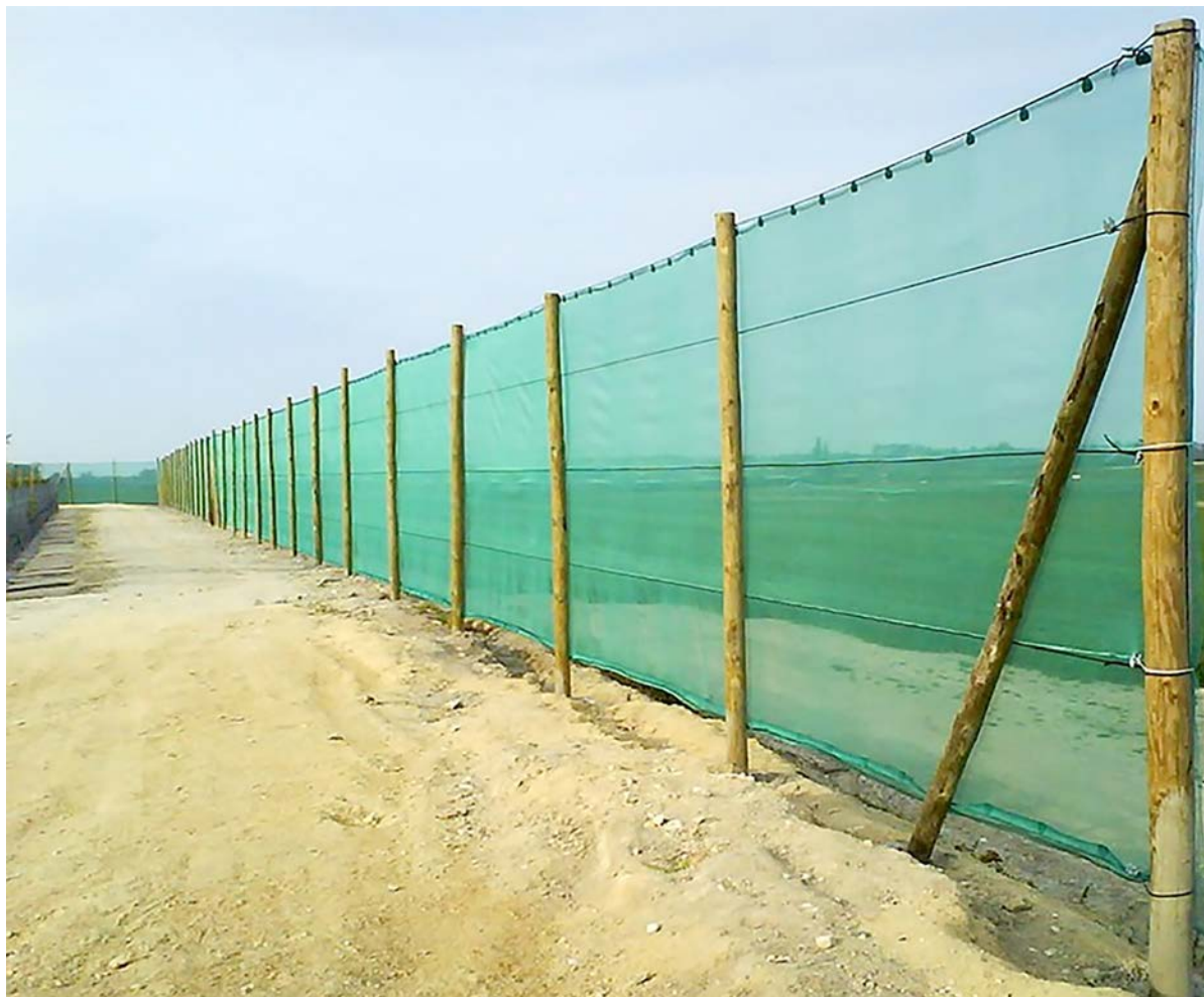
Figure 9 - Sheeting used as a windbreak
