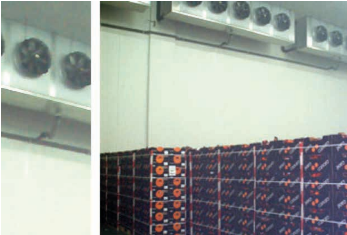
Pre-cooling oranges and clementines in a pre-cooling tunnel, packaged in crates, labelled and placed on disinfected pallets, before being moved to the cold storage room where they will remain until being shipped.
